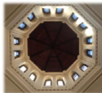
Octagonal church tower, with 16 clerestory windows
