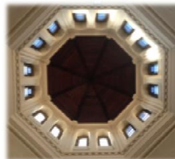
Octagonal church tower, with 16 clerestory windows
